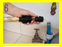
Install the Ferret Head and Outlet Hose to the Ferret and connect them in the usual way to the rising main at POE. For straight forward reassembly use a fitting that will seal over the olive (if used) in the upstream ISV fitting.
