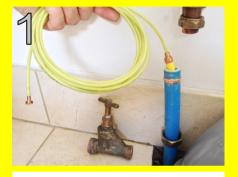
To ensure that the Ferret can be connected at the POE, remove the internal stop valve ISV and use the Head Size and Bend Prover to establish which size of Ferret Head to use and that there are no 90 degree bends fittings.
