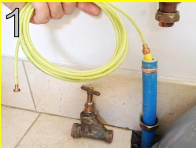
1 To ensure that the Ferret can be connected at the POE, remove the internal stop valve ISV and use the Head Size and Bend Prover to establish which size of Ferret Head to use and that there are no 90 degree bends fittings.
