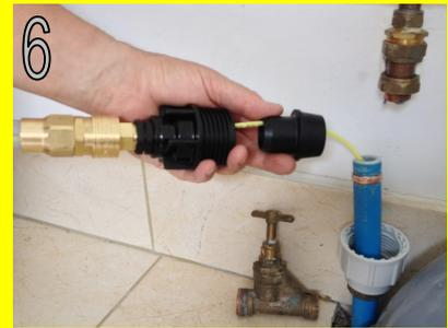
6 Install the Ferret Head and Outlet Hose to the Ferret and connect them in the usual way to the rising main at POE. For straight forward reassembly use a fitting that will seal over the olive (if used) in the upstream ISV fitting.
