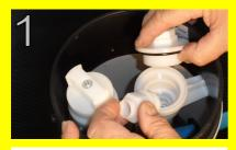
Remove water meter or manifold plug. Then remove the Non Return Valve housing and small "O" ring from the meter manifold. Ensure that the large "O" ring on the water meter manifold is removed and retained for re-fitting later.
